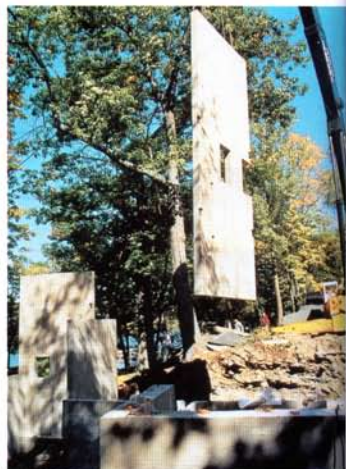
9-10-11. Handling the precast panels in the construction yard; 12-13-14-15. Moving the panels, they are not standard production items, since each has its own original, irregular form.
